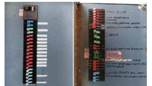
Examples of a Zinsco (Sylvania GTE) panel.
